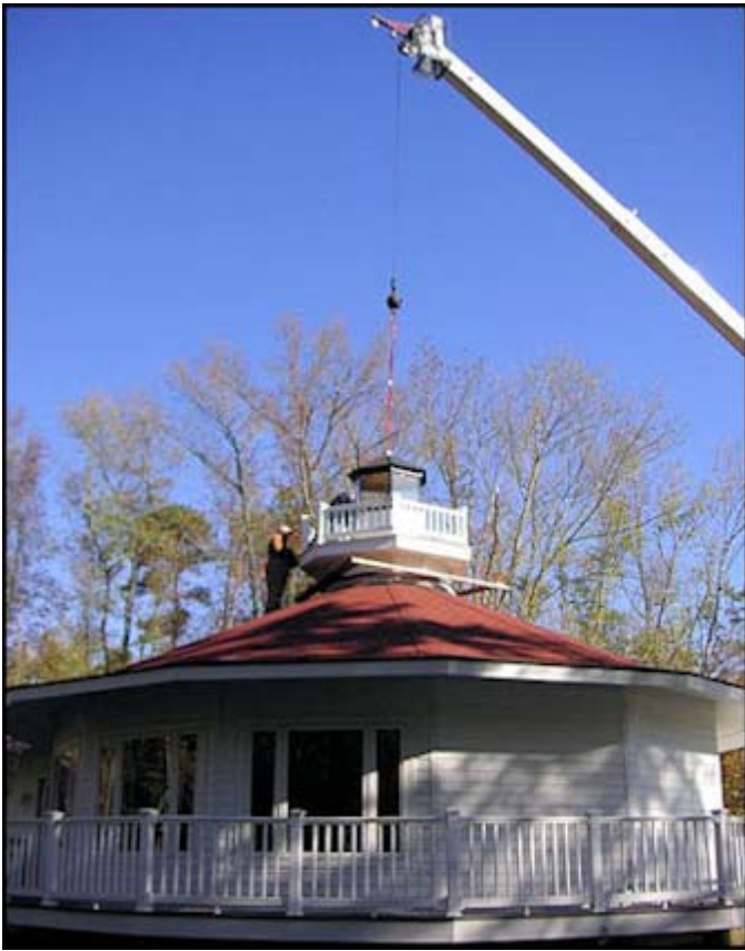
The top is lowered onto the Home of our Own, by Rick's Tree Service. More photos are available on our website @ http://www.uufr-va.com
